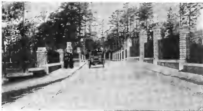
CROSSING THE BRIDGE OVER GEORGIAN COURT.
